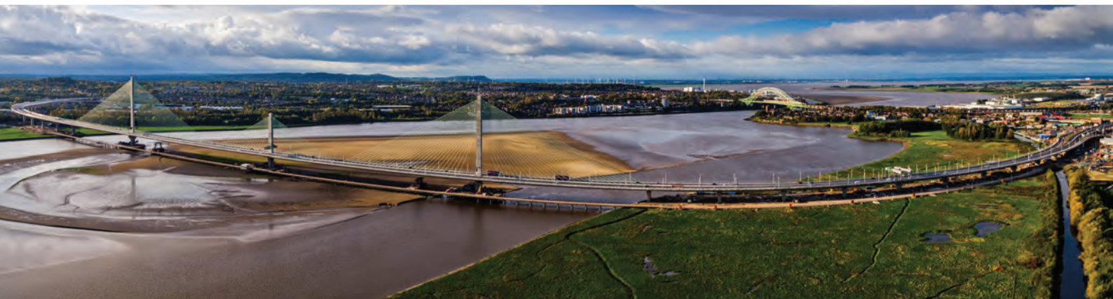
Panoramic view of completed bridge. (All photos: Merseylink Civil Contractors Joint Venture.)
