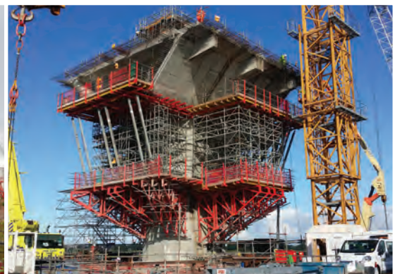
Central pylon pier table. Falsework dismantling ahead of upper pylon construction.
